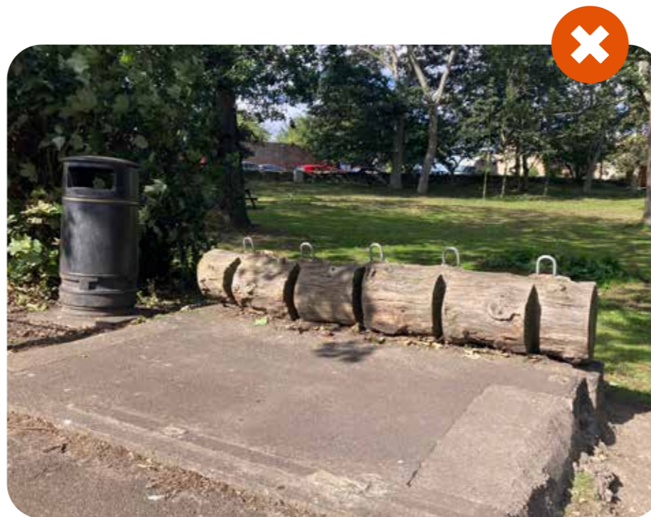
Cycle parking in adapted tree trunk is not fit for purpose
