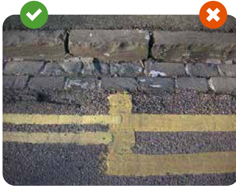
An example of the preferred primrose yellow 50 mm thick lines, alongside traditional yellow lines, Craster
