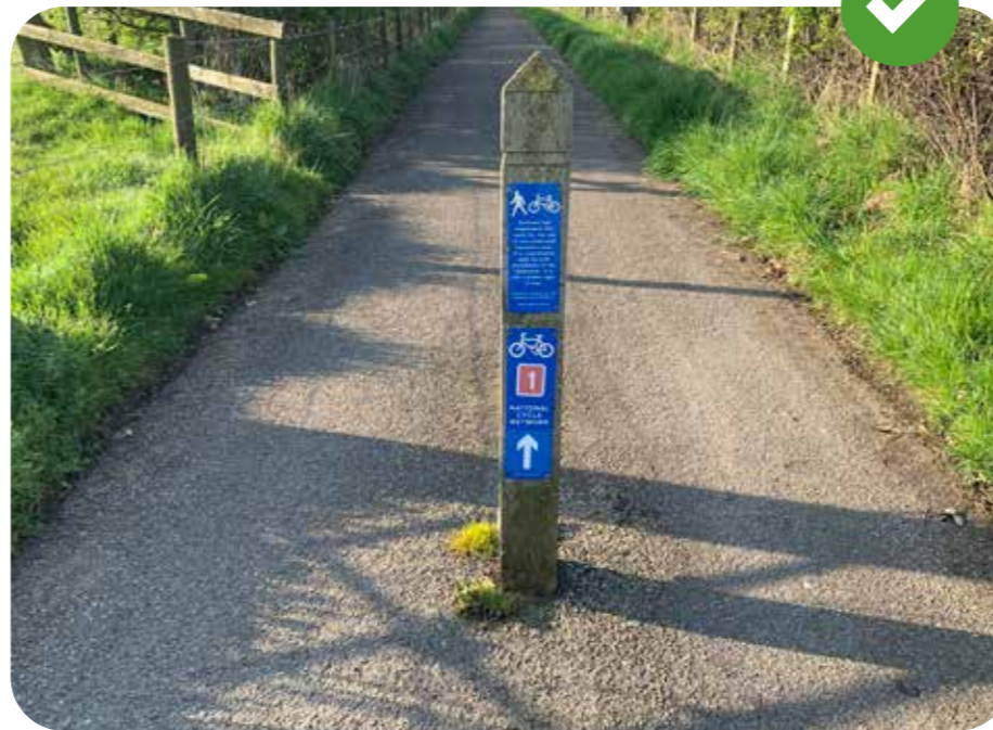
Semi bonded surface provides less visual intrusion within the National Landscape
