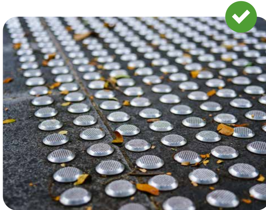
Metal stud tactile paving should be used within the National Landscape
