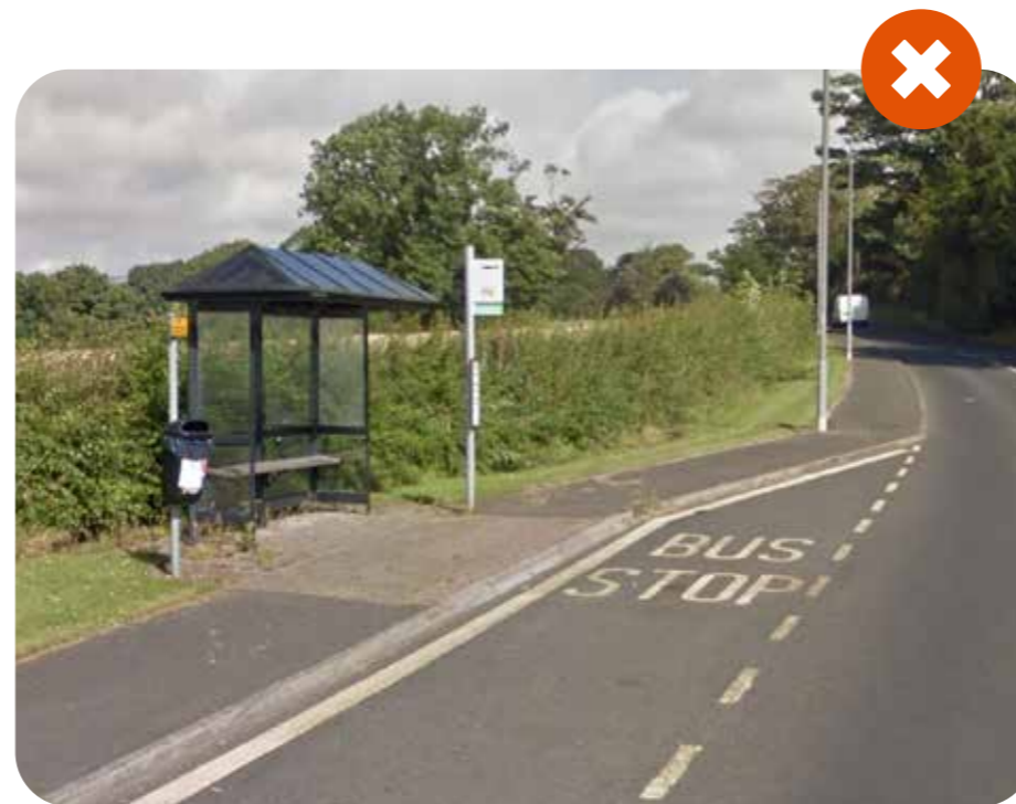
A standard bus shelter, raised kerb, paving and road marking arrangement, Lesbury
