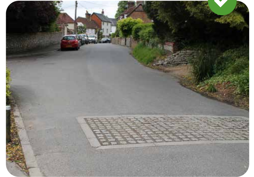
Sensitive traffic calming interventions in Buriton, Hampshire
