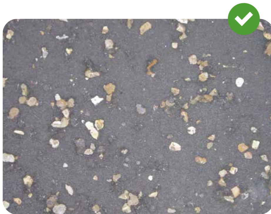
Local aggregates and chippings can be used to articulate key
