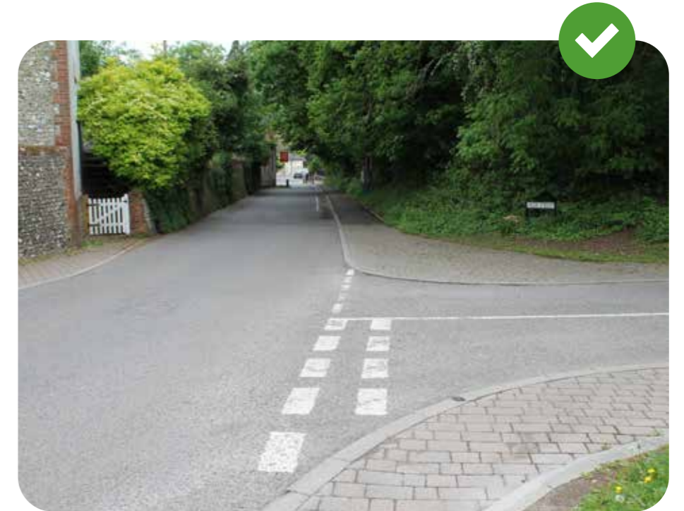
Sensitive use of materials to manage over run for large vehicles
