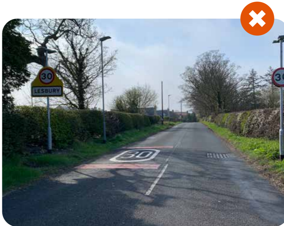
Speed limit signage in Lesbury - Duplication of signage is not required and yellow backing boards should not be used.
