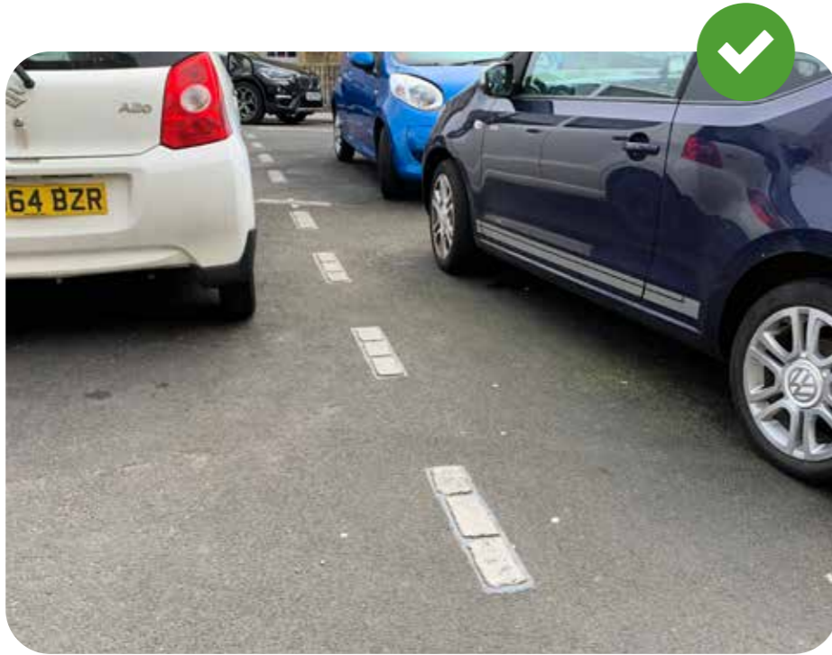
Car parking bays defined with 'quick sett' as an alternative to white lining
