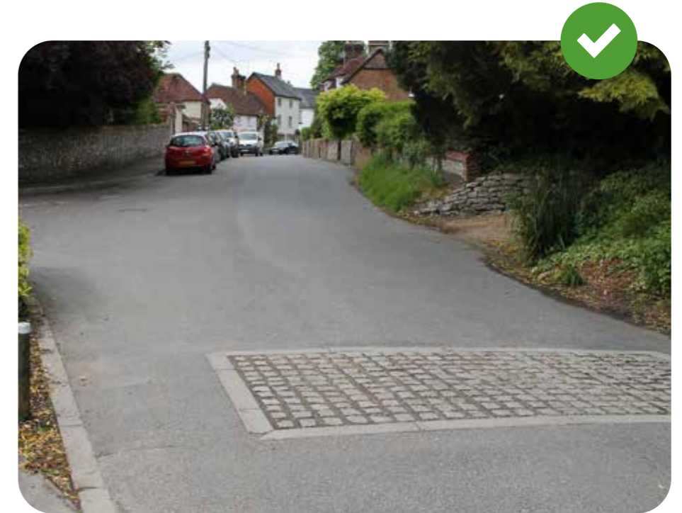
Sensitive traffic calming interventions in Buriton, Hampshire
