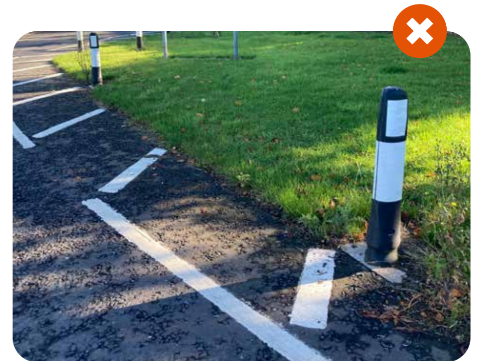
White line markings should not be used at junctions to mark vehicle overrun areas
